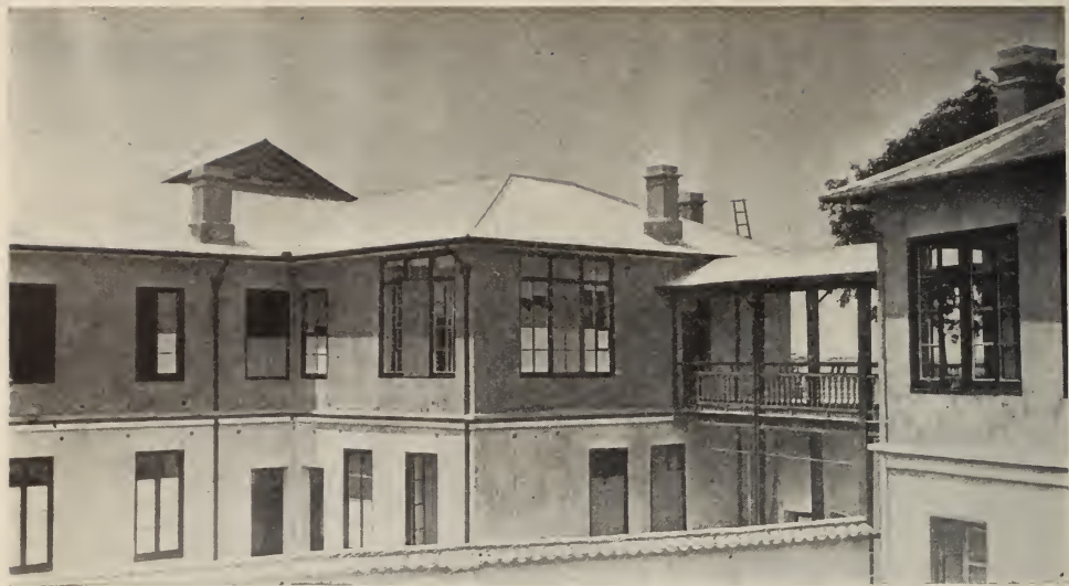
The operating section and covered way connecting it with the Male Ward of the hospital.
